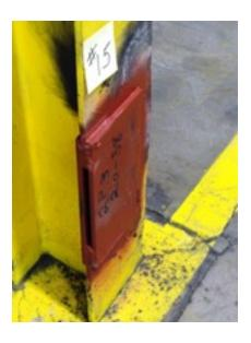
Total column or the bottom to the column replacement occurs when the bend is in the web affects structural integrity. shoring of the roof, cutting or replacement of the column, concrete removal, grout and repairs are part of the process.
