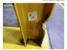
If the flange is damaged, the column can be repaired with flange replacement.
